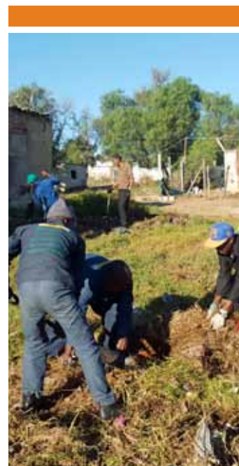
Clearing the area
