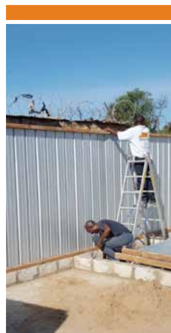
Walls going up
