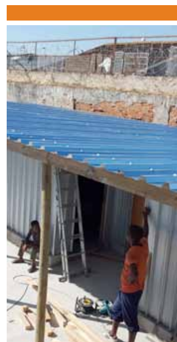
Final work to a toilet block
